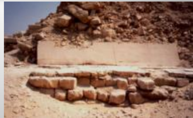
PIT FILLED FOR PYRAMID FOUNDATION
